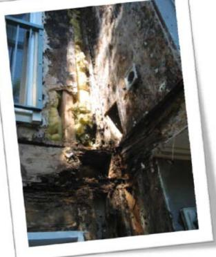
Cobra Construction work closely with the Homeowners Association & Building Envelope Consultant on this complete strip and re-clad of (19) occupied condominium buildings. Substantial rot was uncovered and subsequently repaired. Proper flashings and protective weather resistive barriers were then installed to prevent decay from reoccurring. Costs were carefully tracked and the total construction costs came in approximately \$400K under what was originally budgeted.
