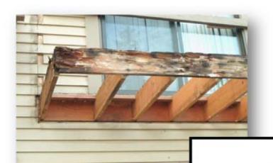
Cobra Construction worked with a local building envelope engineering firm and Homeowners' Association to repair over (70) decks with extensive rot and decay. Repairs included: replacement of rotten framing; re-sloping the decks to create a surface free from standing water; application of new flashings and Pacific Polymer liquid applied waterproofing system; installation of new fascia mounted aluminum railings; venting deck soffits; and painting.
